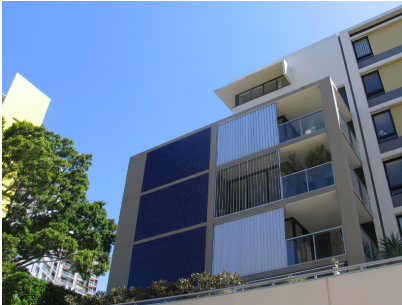
Operable louvres provide climate control
